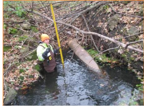
**Figure 4.4-1 Degraded Stormwater Culvert PT2B**
