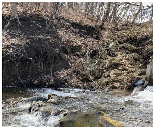
**Right bank erosion downstream of Hwy 5 culvert**
