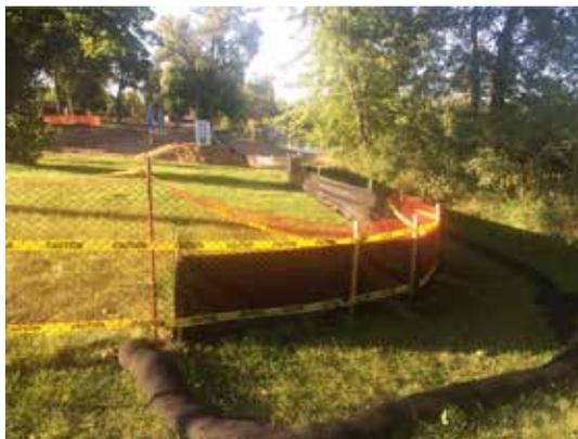
*Temporary and permanent erosion control measures are essential to reducing pollution in runoff*
