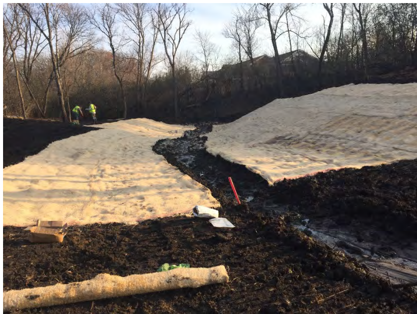
Installation of erosion control blanket on areas where grading was finished.
