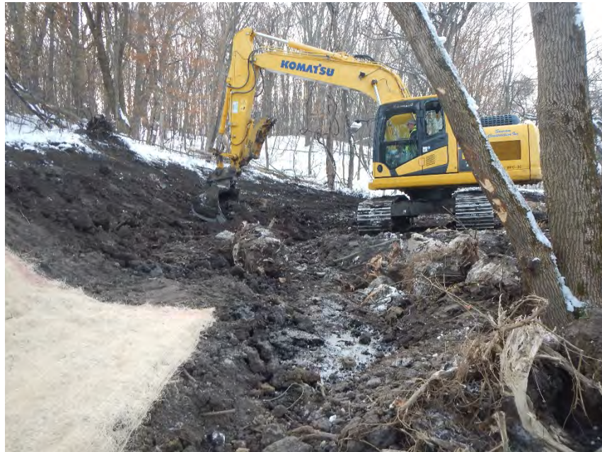
Installing root wads toward the upstream end of the project
