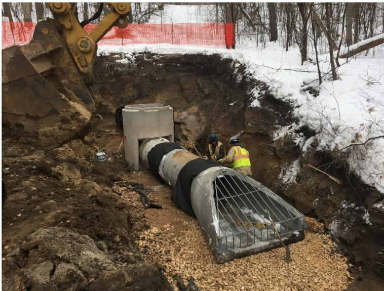
**Installation of a storm sewer toward the downstream end of the project**
