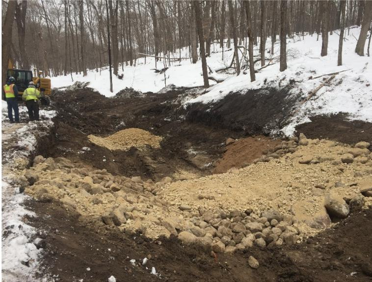
**Beginning installation of a rock riffle toward the upstream end of the project**
