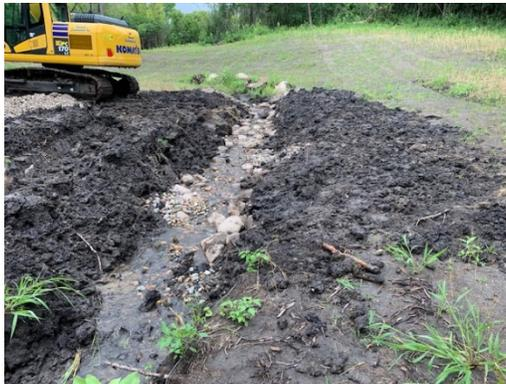
*Additional Rock Riffle being install where head-cut began forming this spring*
