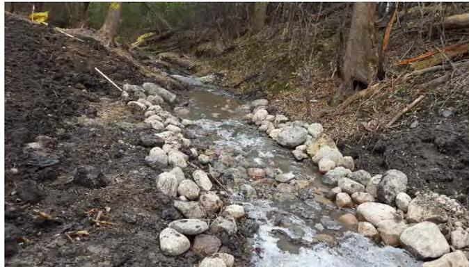
**Flow through a newly constructed rock riffle at the downstream end of the project**
