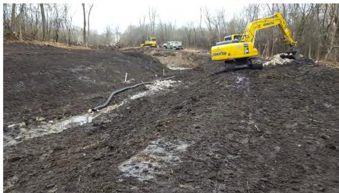
**Grading and installing another rock riffle. Note the pipe being used to pump water around the active work area.**
