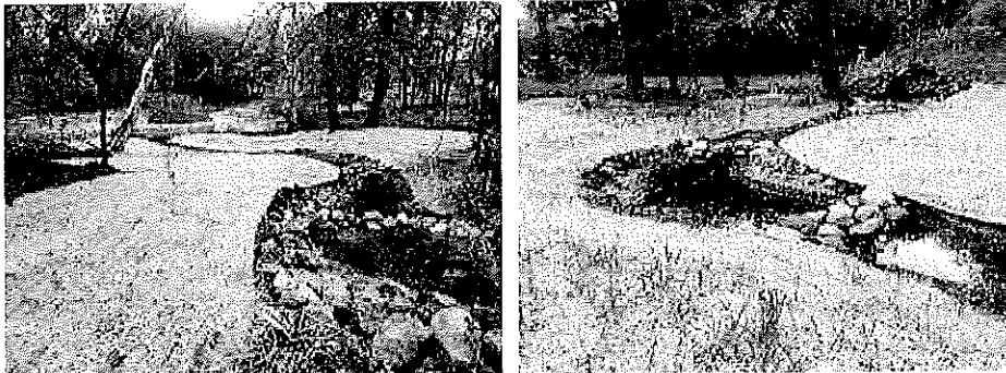
Newly seeded and stabilized swale with rock riffles
