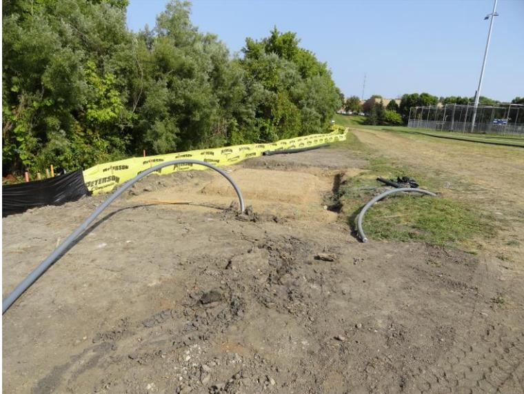
**Pump pad foundation (has since been re-excavated to remove additional subgrade soils) and directionally drilled HDPE.**
