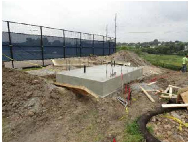
**Photo of the water treatment shelter foundation, after forms removed**
