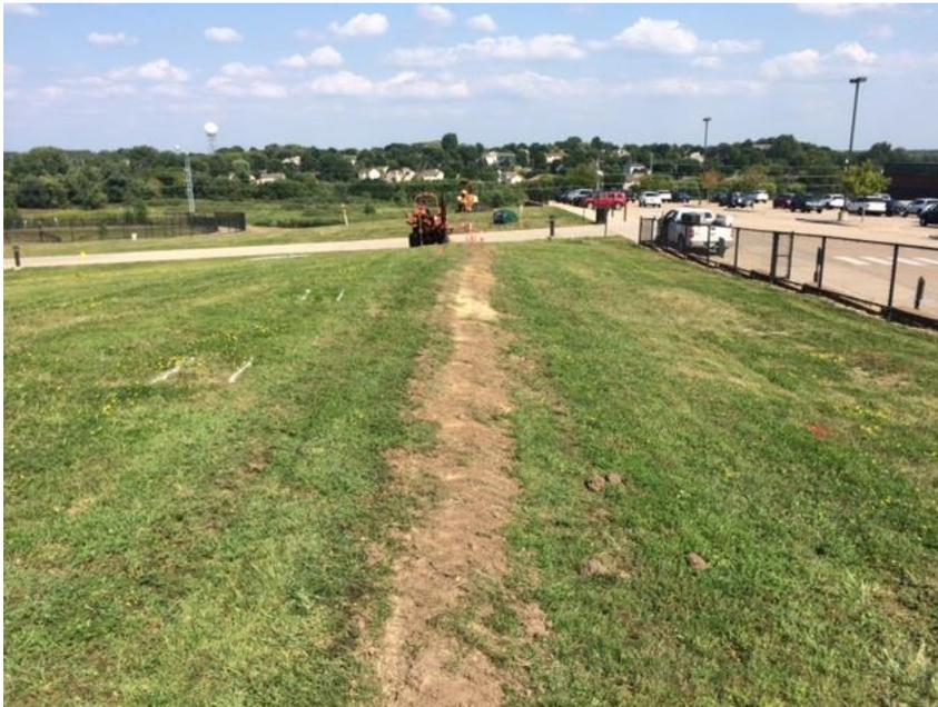
**Low voltage communication line in Magellan Easement from treatment shelter to existing irrigation box/controls**
