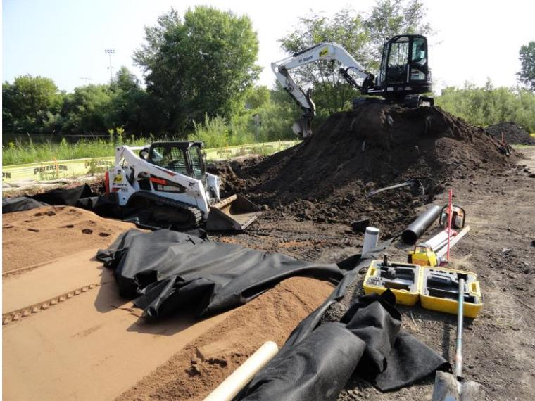
**Iron-enhanced sand filter excavation.**
