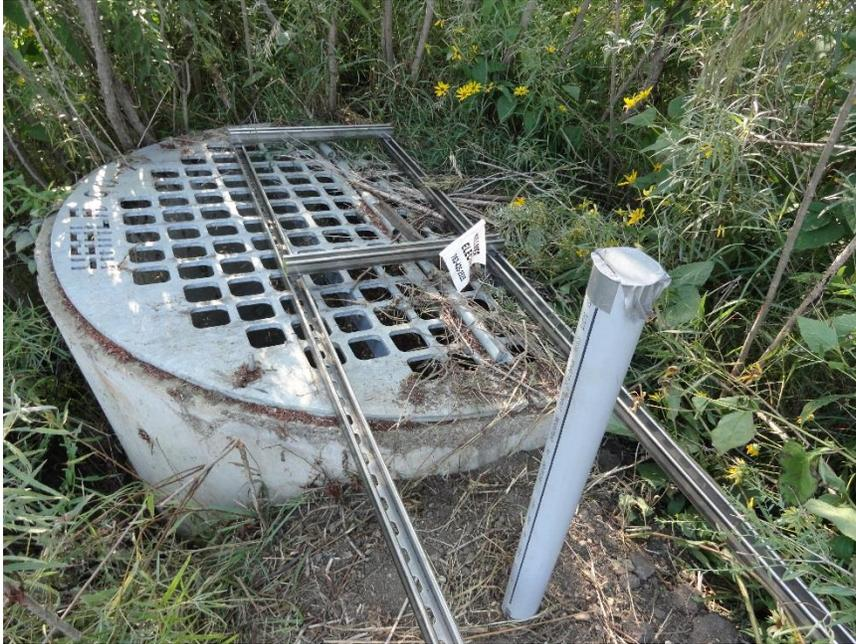
**Line for water level sensor at existing pond outlet structure**
