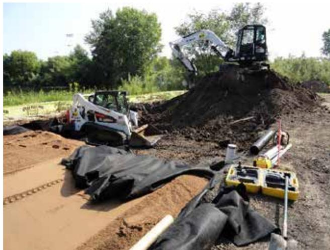
**Photo of the iron enhanced sand filter installation**
