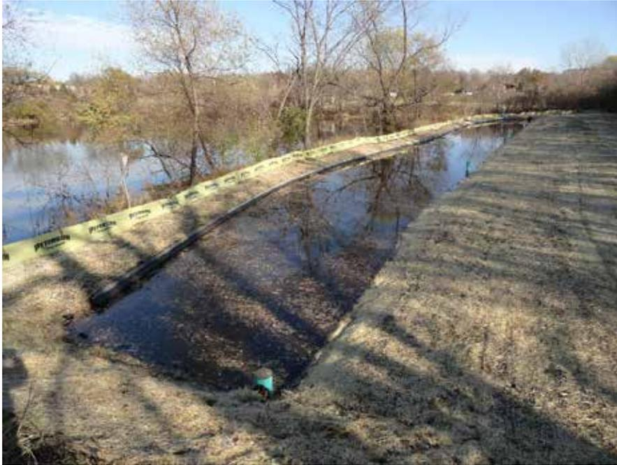
**Completed iron-enhanced sand filter during start-up/testing**
