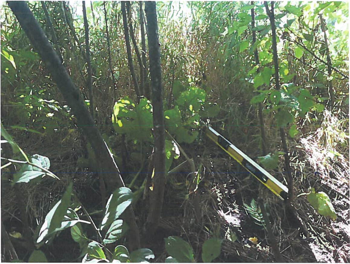
Picture 3: North side of box culvert, east bank of Riley Creek (Existing slope – 2.4H:1V)
