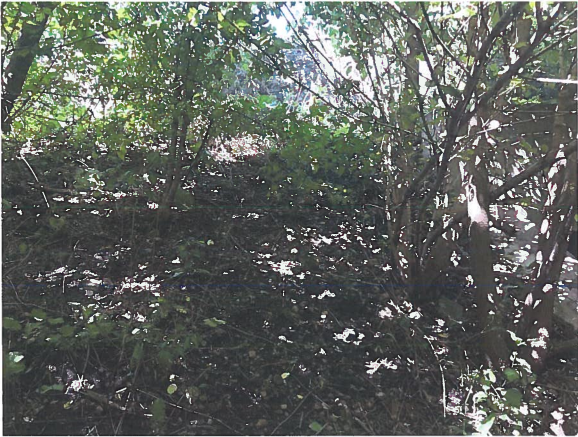
Picture 5: South side of box culvert, west bank of Riley Creek (Existing slope – 1.8H:1V)
