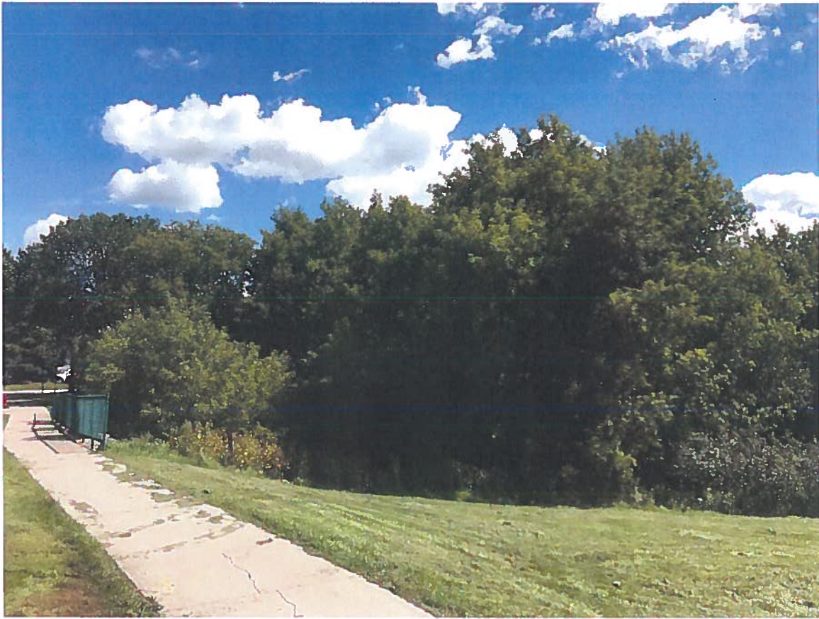
Picture 1: South side of box culvert – mature trees and existing vegetative cover
